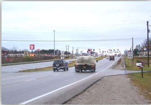
US 25E between MP 25.400 & 25.600, looking northwest
