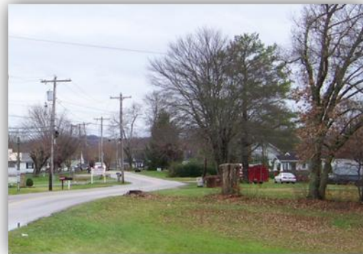
KY 312 at MP 1.700- 1.800, looking east
