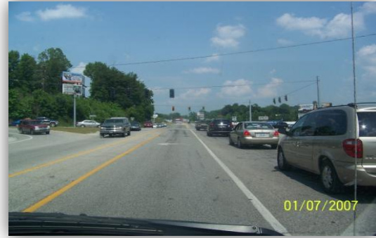
US 25 & US 25E Intersection at south leg, looking north
