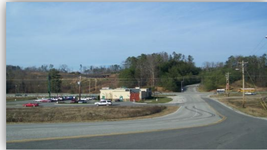
Arena Dr. at US25W Int., looking north on Hospital Ent.
