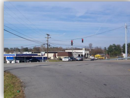
US 25E/KY 3431 Signalized Int. looking North on KY 3431
