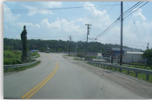
KY 3431 near KY 1223 & US 25E Int., looking south
