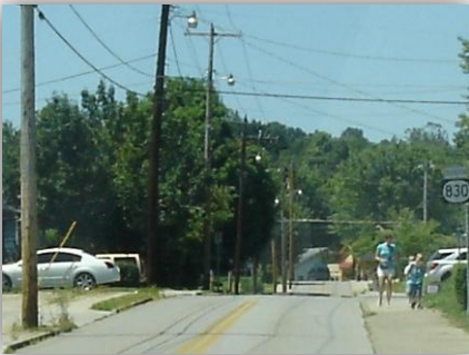
KY 830 between KY 312 & Engineering St. Int., Looking North
