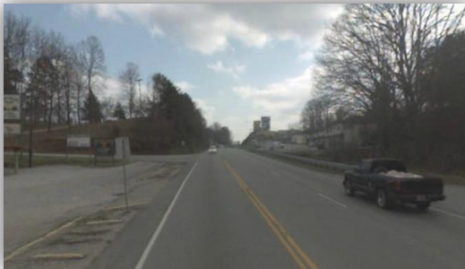
Near US 25 & KY-2392 Int. at MP 0.800, looking South
