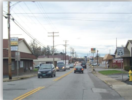
US 25W north of US 25W & KY26 Int., looking north
