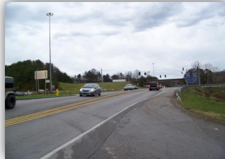
US 25W at mile point 29.5, looking east upon Interstate 75
