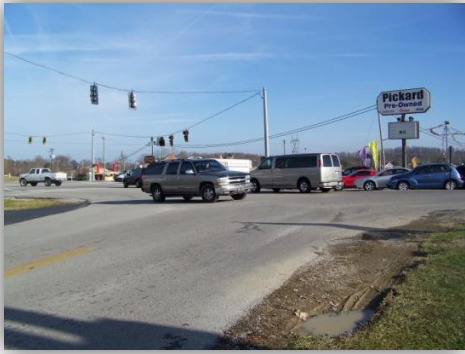
KY 1629 at N. Commonwealth Road Int., looking north
