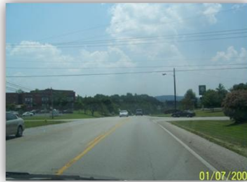
Looking south on KY 312 near N. Commonwealth Ave. Int.
