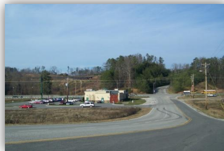
Arena Dr. at US 25W Int., looking north on Hospital Ent.
