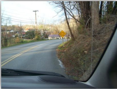
KY 727 near Woodland from MP 3.300 to 3.500, looking east
