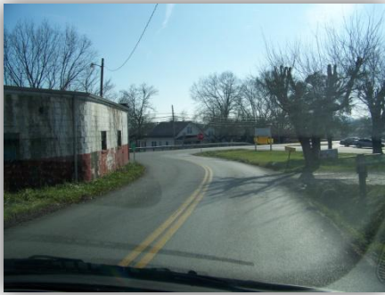
KY 3431 approaching US 25W “Y” Int. looking south
