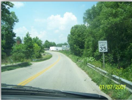
KY 3431- looking north on MP 1.000 to 1.200
