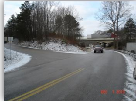
Looking West from KY 727 onto KY 1259 on left with I-75 Bridges in the background on the right.
